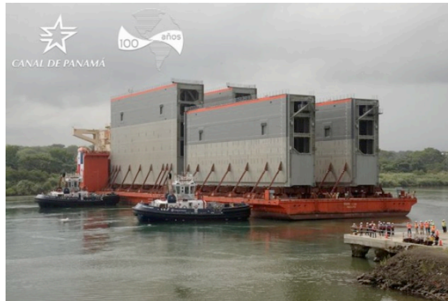
Exhibit 6. Panama Canal rolling gates for new lock chambers 36
